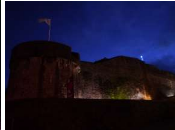
Dramatic night-time lighting
